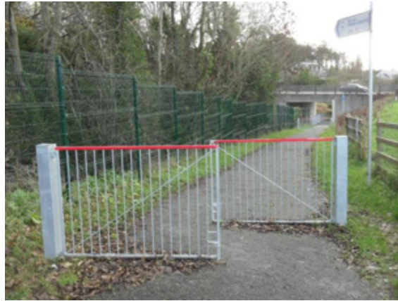
Figure 13: Staggered gates prevent unauthorised vehicular access. The gates can be opened on request for events with large footfalls.
