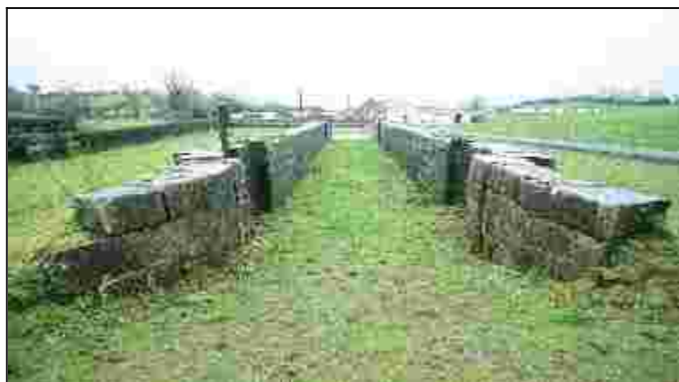
Fig 4.1 Partly infilled lock chamber at Templetate (lock 22).
