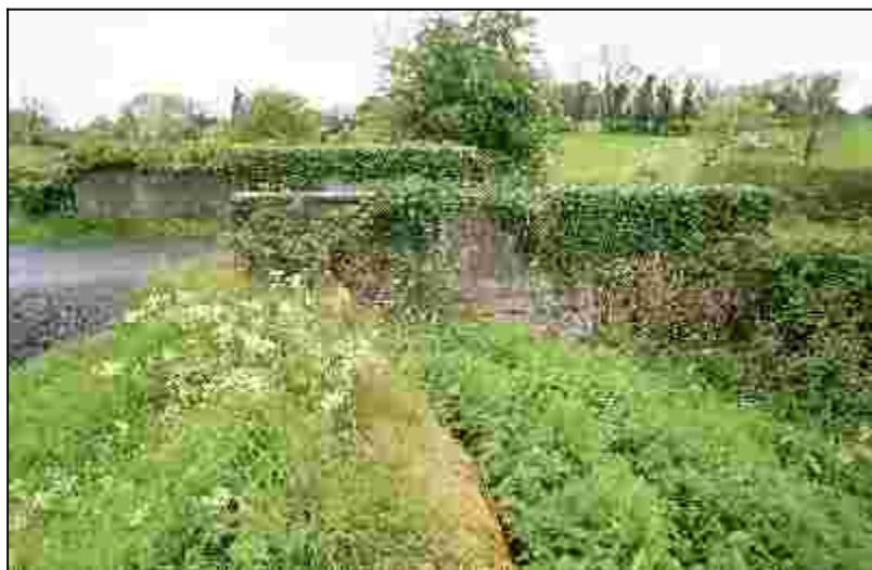
Fig 4.19 The original swing bridge at Drumsloe near Clones (2421) has been replaced with this concrete culvert bridge.
