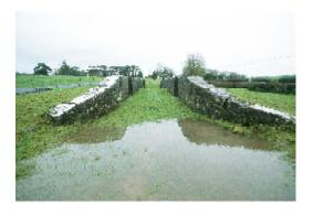
2201\_04 FWH 08/01/2008 Land sluice mechanism housing and stop plank groove at west side of top end of lock.
